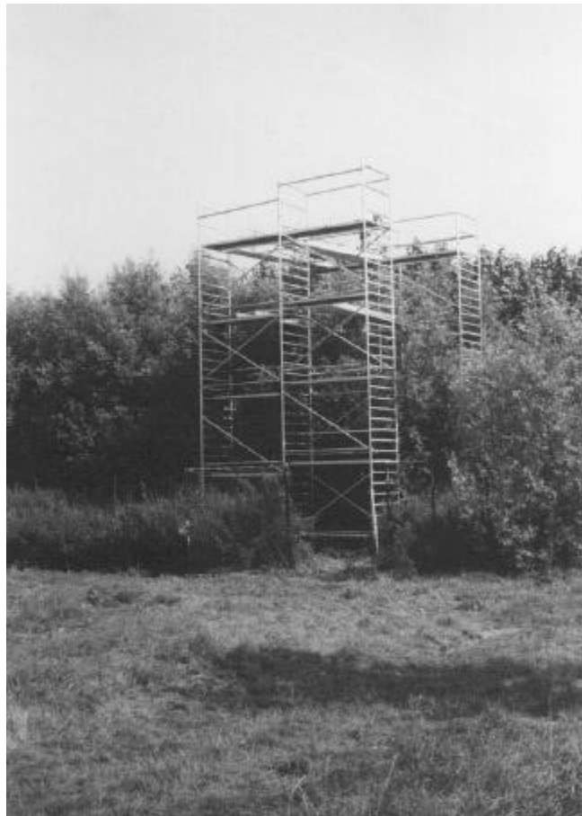
Fig. 2. Scaffolds joined by gangplanks erected around the Salix fragilis L. tree
