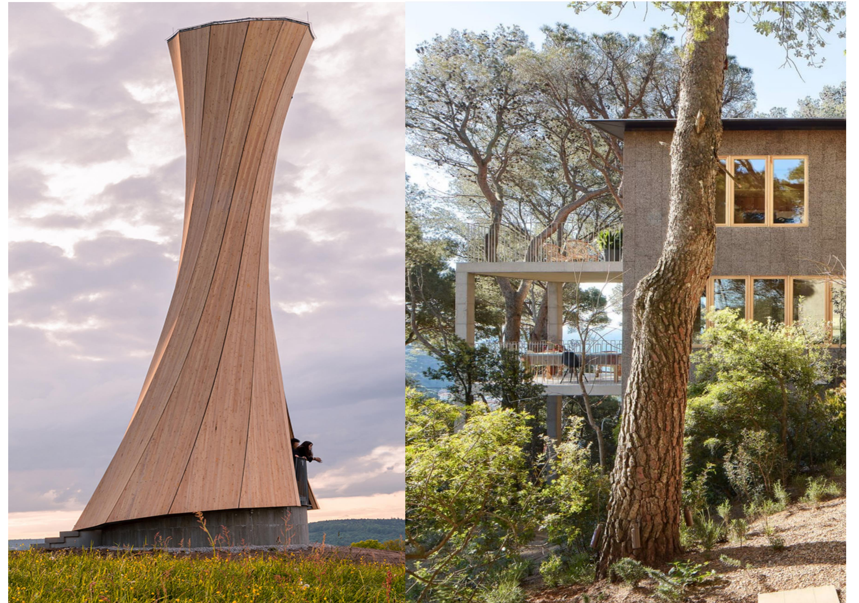
Left: Urbach tower, Germany. The curved timber components that give the tower its unique structure were designed and produced as flat panels that deform autonomously into predicted curved shapes when dried. © ICD/ITKE. Right: House with cork as exterior cladding © José Hevia
